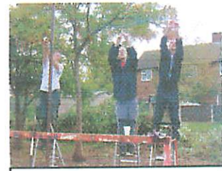
Repairing the fence
